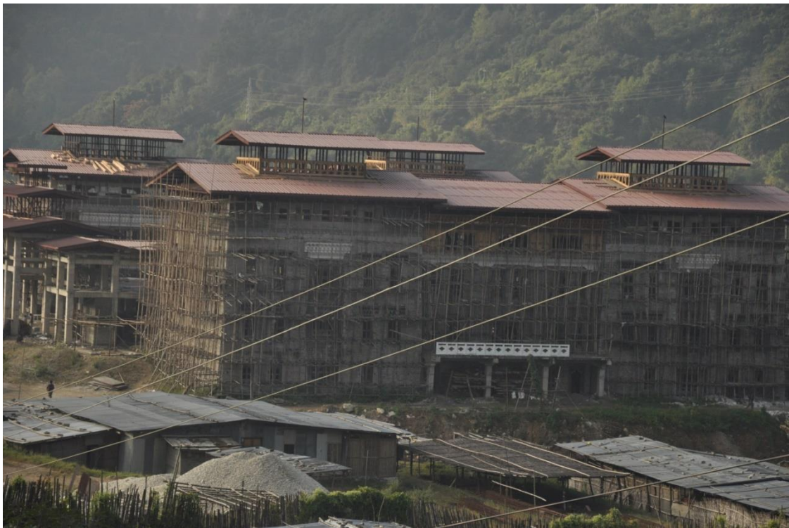
Figure 4: view of the Dzong showing blocks C,D and E.
