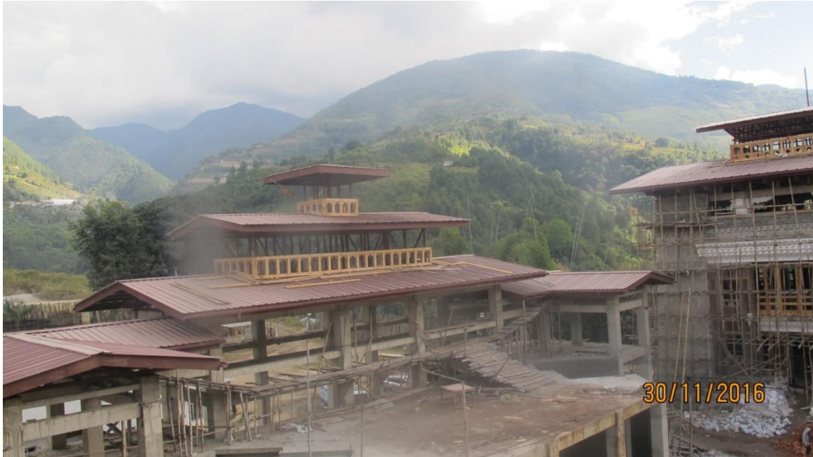
Figure 3: View of the Entrance Foyer, block D.
