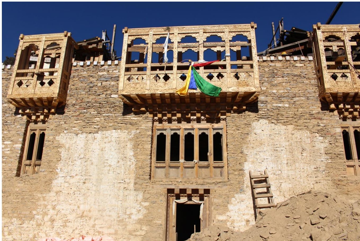
Fig 2: Renovation works on Wogmin Lhakhang in progress.
