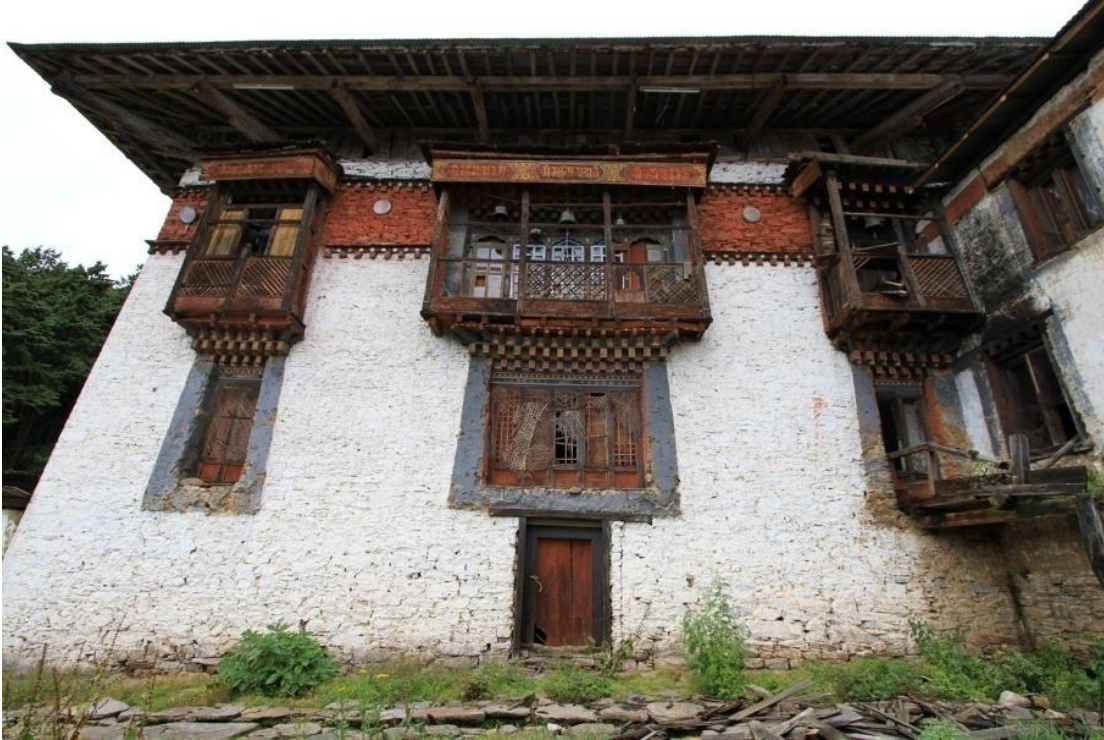
Fig1: Wogmin Lhakhang before the renovation works.
