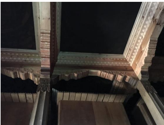
Fitting & Fixing of Kikhor Planks
