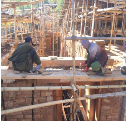
Construction of CRM Wall in mud mortar up to 1 st floor level completed
