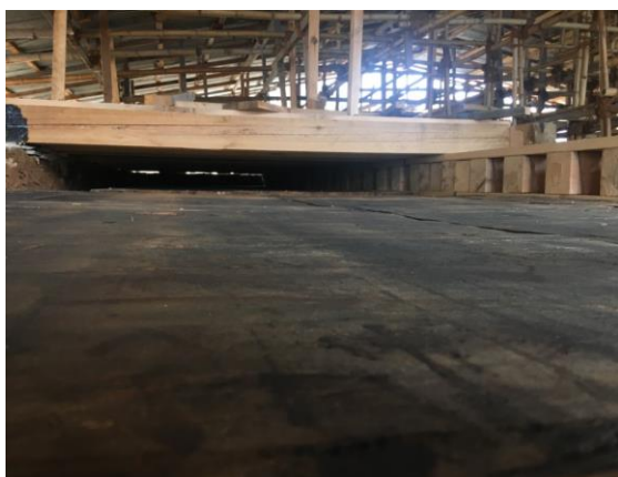
Fitting and fixing of battens, cham and planks for main lhakhang
