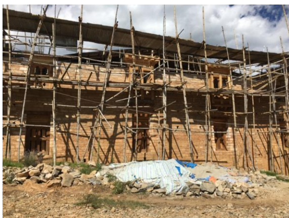
Fitting and fixing of timber component including Gayka, Window, Door & Rabsay completed up to 1 st floor level
