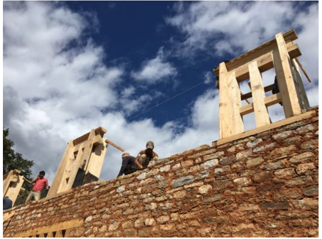
2. Laying out the Gedkar on the first floor.
