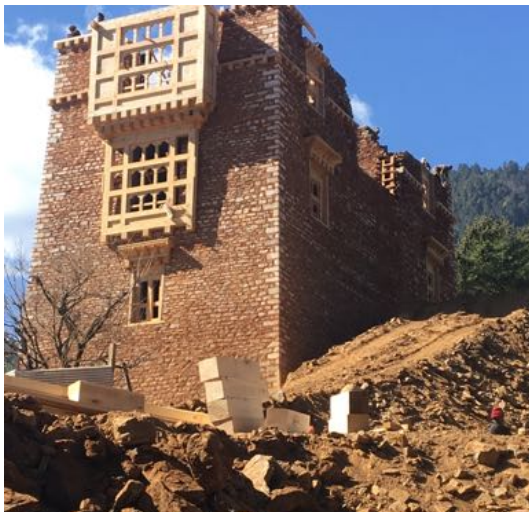
5. Construction of the third floor level in progress
