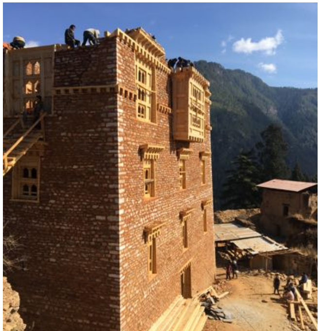
6. Construction of the rabsey in the third floor.
