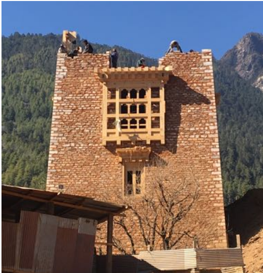
4. Completion and Placement of the Rabsey on the second floor.
