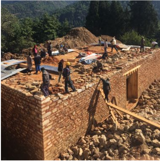
1. Completion of the ground floor level
