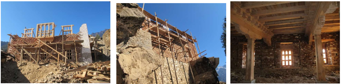
Figure 4: Dasho Dzongda's Office block- under renovation
