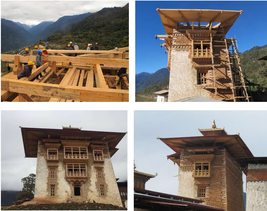
Figure 3: Utse renovation work
